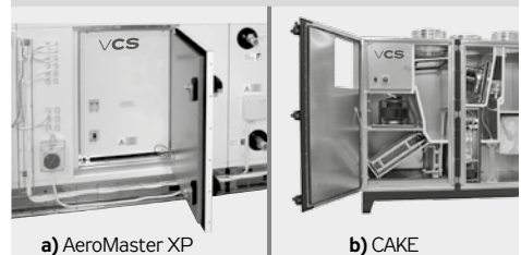
Figure 2 – installation inside air handling unit
